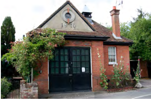
Old Fire Station 1910 roughcast first floor above surviving doors; shingled roof
